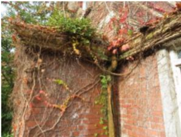
Figure 23: Current state of the drainpipes (Branford, 2020, p19)
