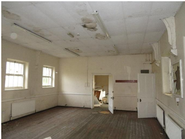
Image 9, Suspended Ceilings Showing condensation staining. (Branford, 2019)
