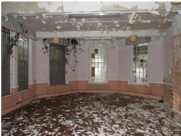
Image 18, Decoration decay attributed to poor ventilation and condensation (Branford, 2019)
