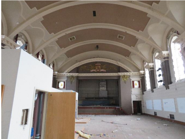
Image 11, Vaulted fire-proof concrete ceiling (Branford, 2019)
