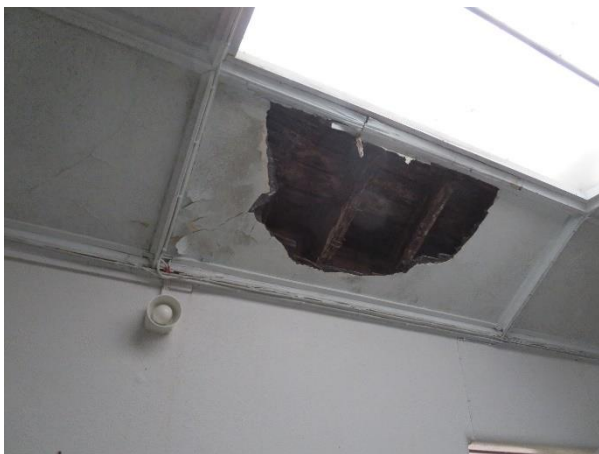
Image 2, showing area of ceiling decay attributed to roof defects (Branford, 2019)
