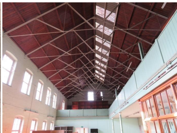
Image 6, Roof structure of store (Branford, 2019)
