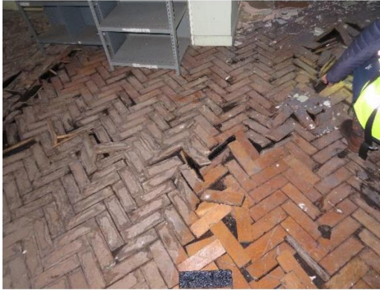
Figure 8 Parquet flooring has been damaged by water ingress (Branford 2020, p. 13).
