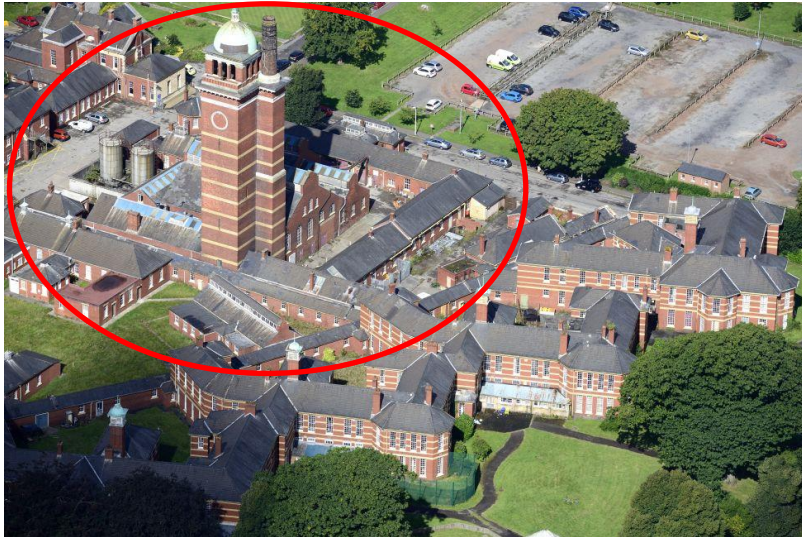
Figure 21: The former Water Tower and its adjacent buildings (highlighted) will become a Climbing & Adventure Centre. (Photograph courtesy of RCAHMMW. 26 th August 2016)
