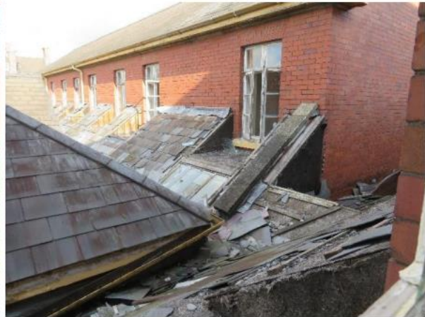
Figure 7 Damage to roof areas is visible throughout the site. A lack of ongoing maintenance, lead theft and general vandalism being the general cause (Branford 2020, p. 12&13).
