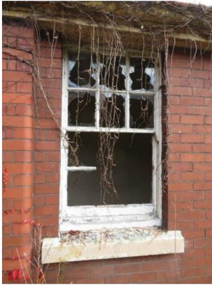
Figure 6 Extensive damage to timber and glazing is visible throughout the site as a result of vandalism which has facilitated water and vegetation ingress throughout the site (Branford 2020, p. 30).
