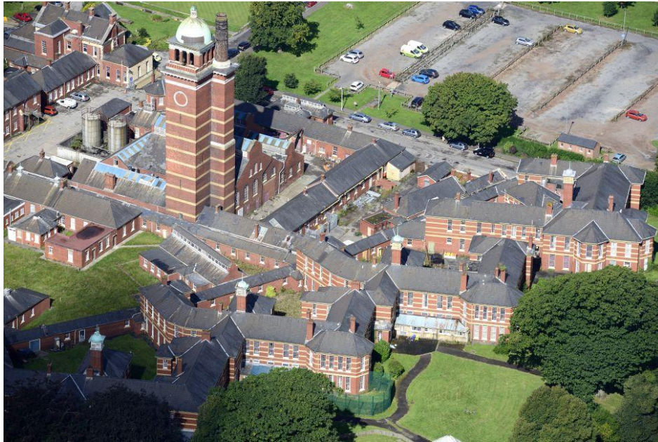
Figure 3: The Hospitals 150ft Water Tower dominating the hospital site. The hospital incorporates 10 self-contained wards for 750 patients but with capacity for 1250 (Morris 1965, p. 9). (Photograph courtesy of RCAHMW. 26 th August 2016)
