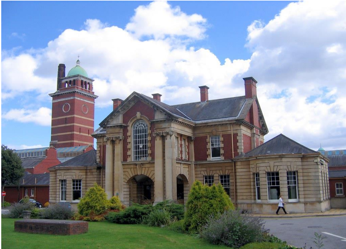
Figure 20: Former Administration Building to be retained as primary entrance to the Creative Quarter. A Community Hub will provide community spaces and uses will re-connect the local community to the building. (Photograph courtesy of https://www.flickr.com/photos/roath_park_mark/239113702 )
