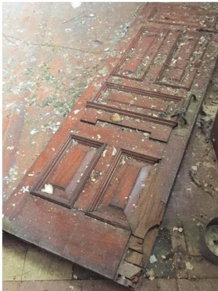
Figure 9 Many original internal fixtures and fittings remain including an original door which has been removed from its hinges and vandalised (Branford 2020, p. 36).
