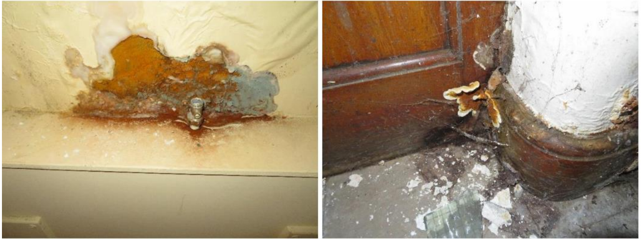
Figure 10 Evidence of wet rot is visible internally as a result of extensive ongoing water penetration (Branford 2020, p. 37).
