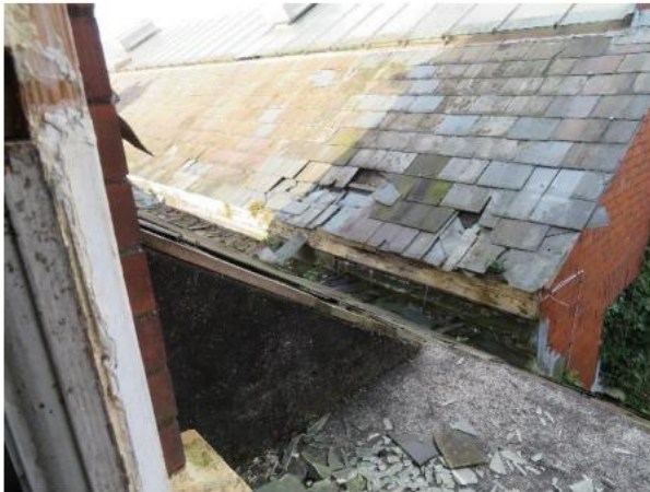
Figure 7 Damage to roof areas is visible throughout the site. A lack of ongoing maintenance, lead theft and general vandalism being the general cause (Branford 2020, p. 12&13).
