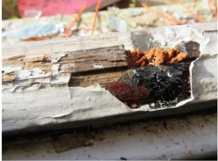
Figure 6 Extensive damage to timber and glazing is visible throughout the site as a result of vandalism which has facilitated water and vegetation ingress throughout the site (Branford 2020, p. 30).
