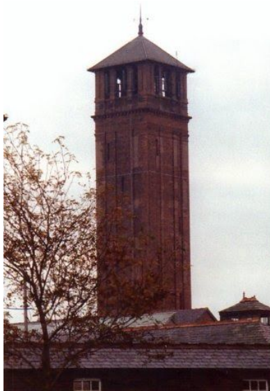
Fig. 10. The water tower of Winwick Hospital (destroyed)
