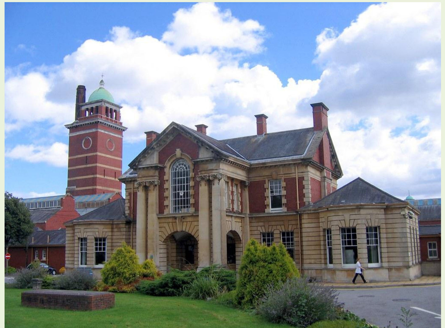
Figure 12: Main Entrance Building (with Water Tower to rear), Whitchurch Hospital. Source: www.flickr.com/photos/roath_park_mark/239113700
