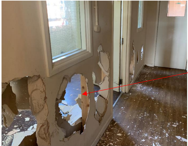
Figure 15: Damaged walls (Zhang, 2019)
