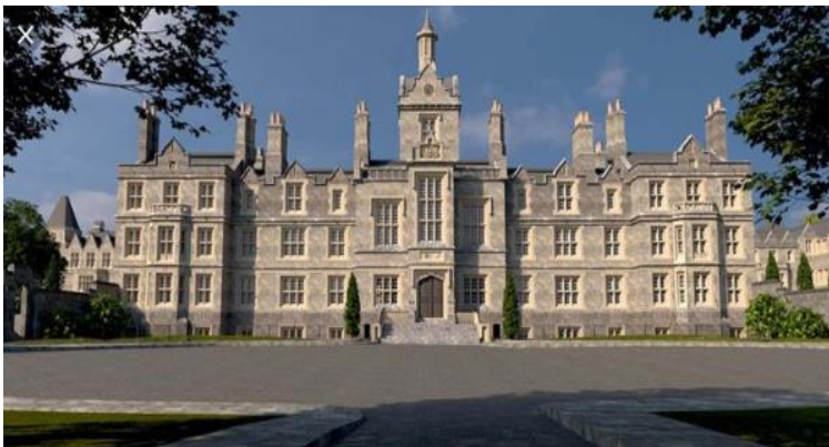
Figure 20: Denbigh Hospital – prior to extensive damage (Kenwright L, 2018)
