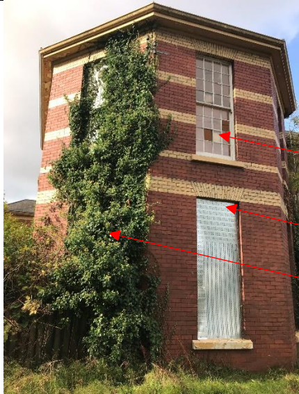
Figure 16: Steel grids at ground floor. (Adams, 2019)
