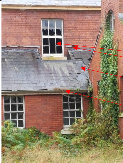
Figure 17: Slipped Slates and missing lead (Adams, 2019)
