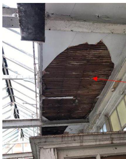
Figure 12: Fallen plaster work & exposed lath (Adams, 2019)
