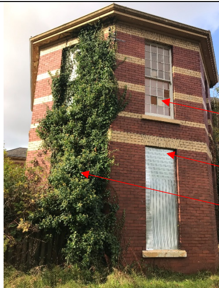
Figure 15: Steel grids at ground floor. (Adams, 2019)
