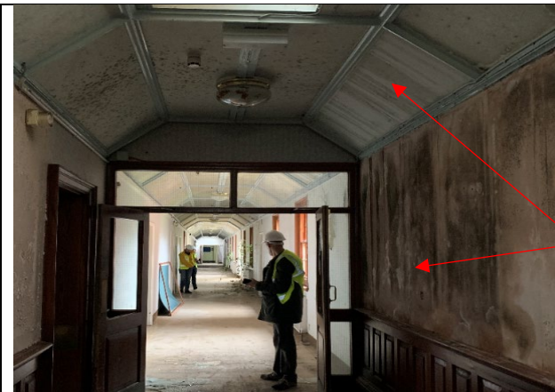
Figure 13: Damp corridors (Zhang, 2019)
