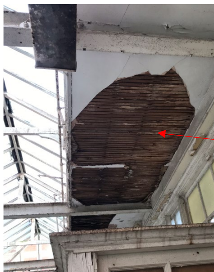
Figure 11: Fallen plaster work & exposed lath (Adams, 2019)
