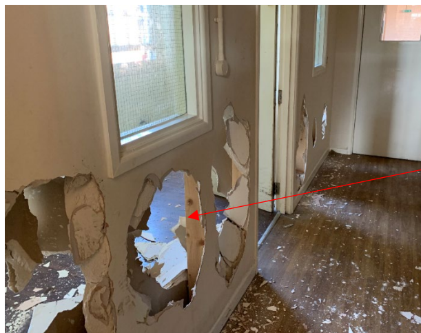
Figure 14: Damaged walls (Zhang, 2019)
