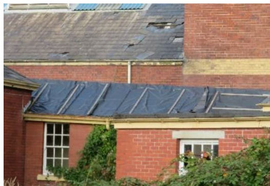
Figure 16: Failed roof surface covered with plastic sheet (Branford P, 2020)
