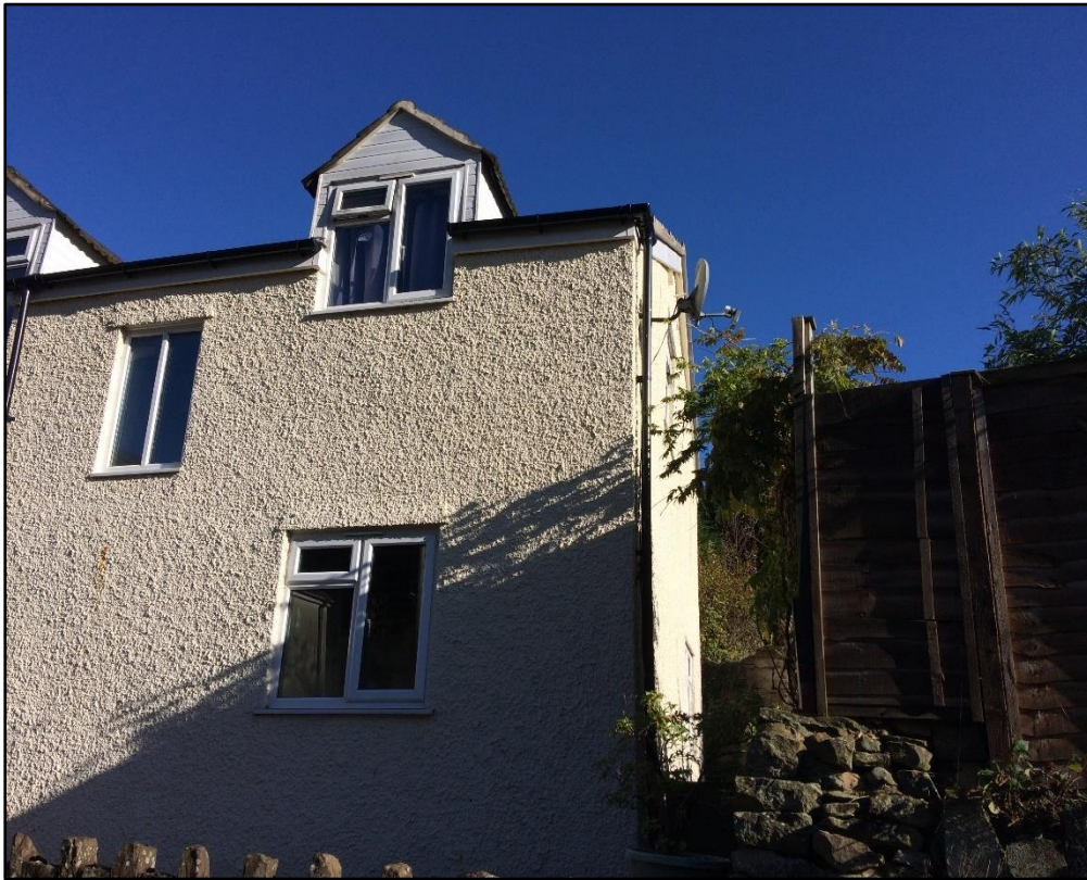
Figure 33: Traditional stone-built cottage renovated with hard non- permeable cement roughcast render applied externally (Source: Gwynne, 2017).
