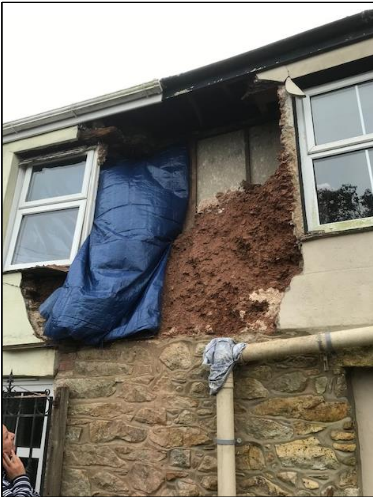
Figure 39: Collapse of the cob wall (Source: Gwynne, 2019).
