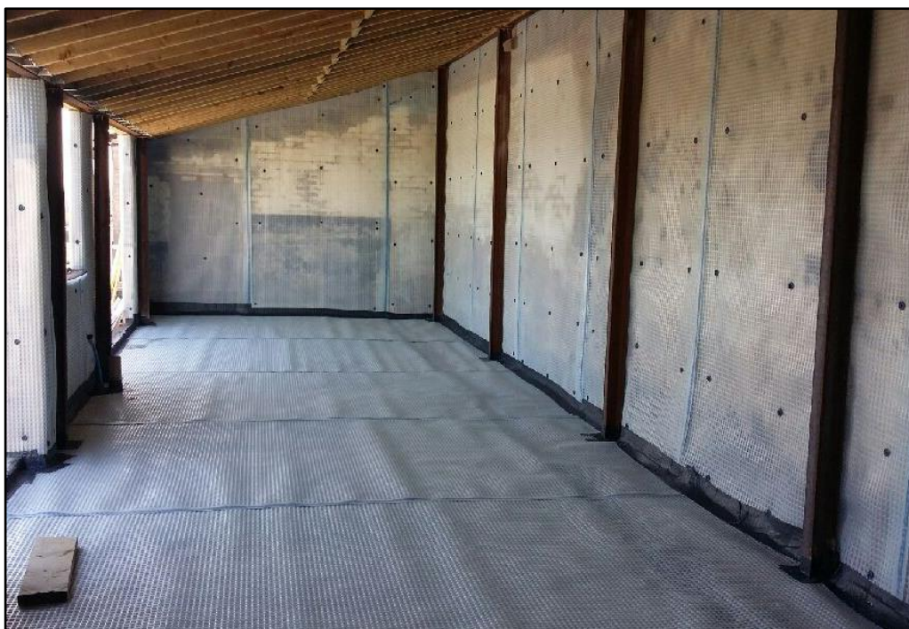
Figure 31: Tanking system fixed to top of original floor and internal face of solid walls (Source: Gwynne, 2018).
