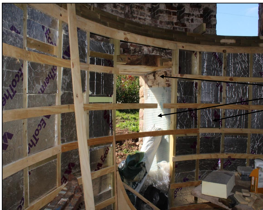
Figure 20: Upgrading of solid walls with modern non-vapour permeable tanking membranes and high density polyisocyanurate insulation board
