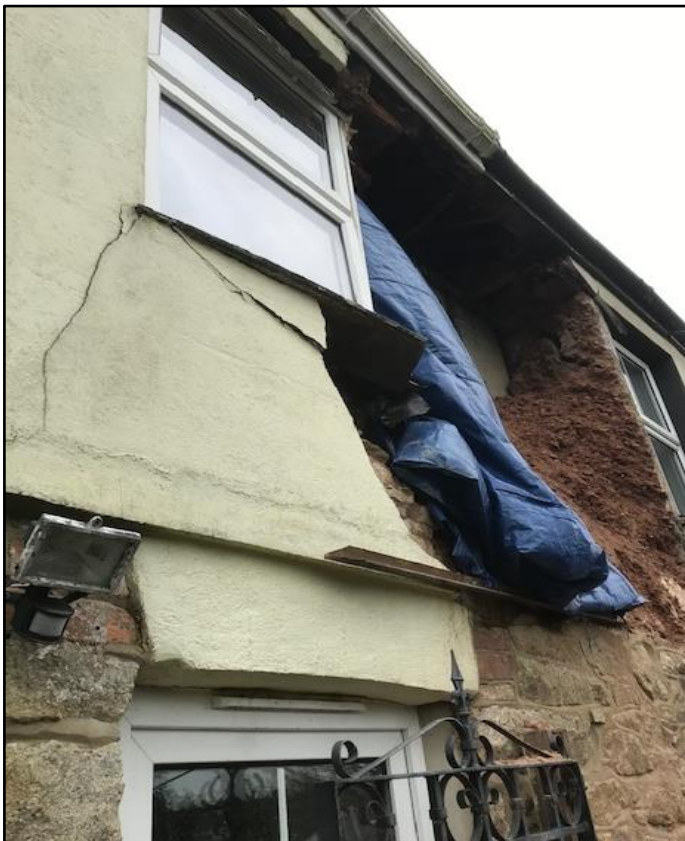
Figure 38: Collapse of the cob wall (Source: Gwynne, 2019).
