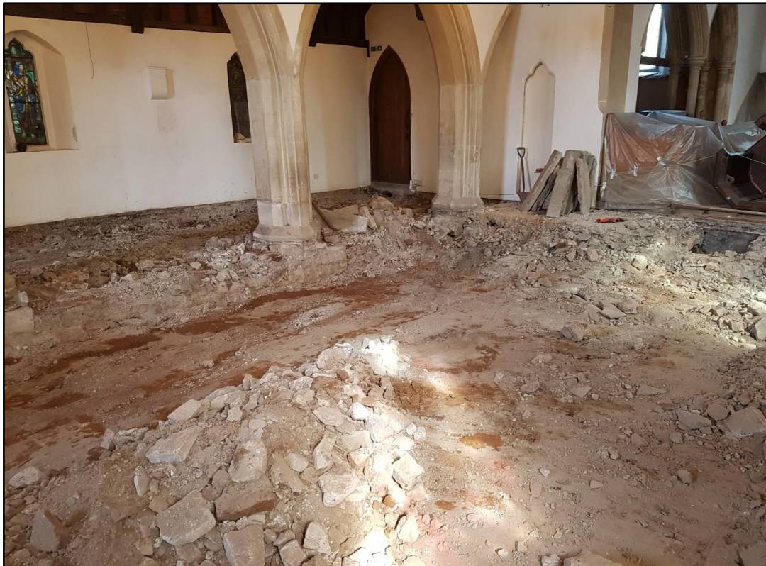
Figure 24: Hardcore being laid (Source: Gwynne, 2019).
