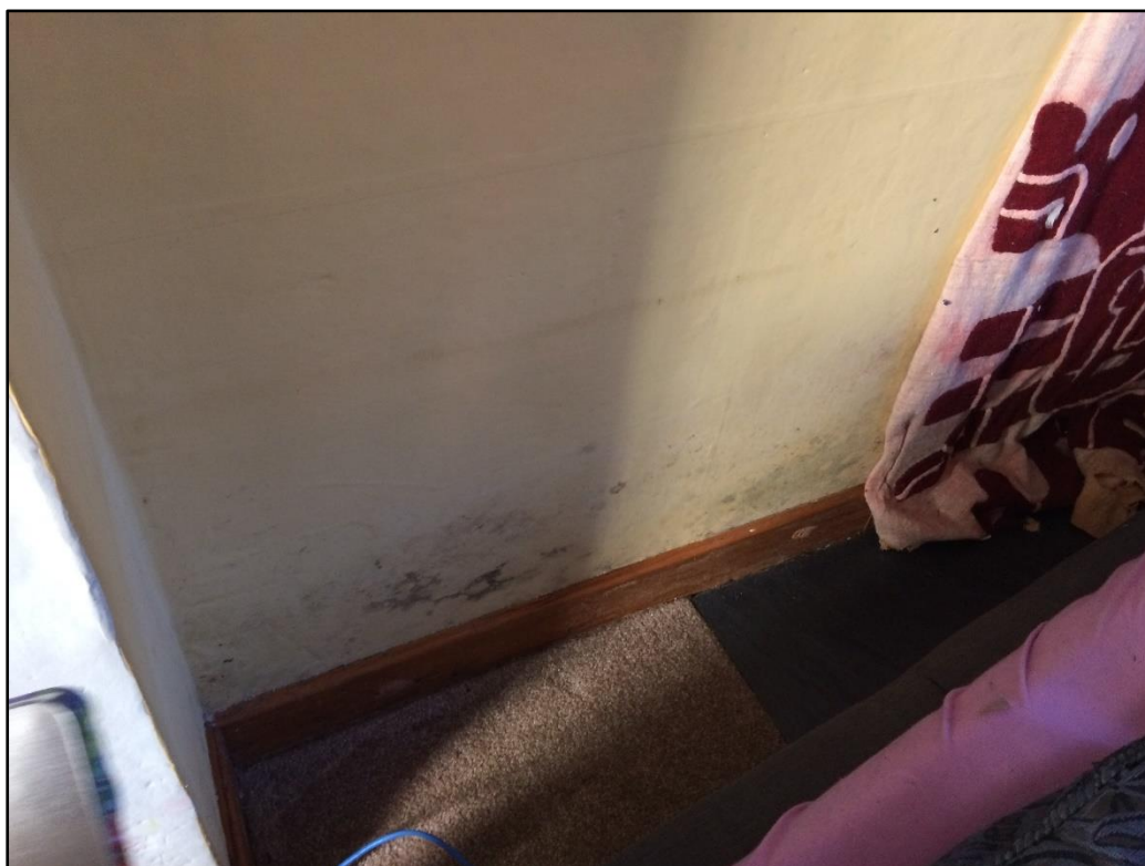
Figure 36: Black mould growth evident on internal plaster finishes (Source: Gwynne, 2017).
