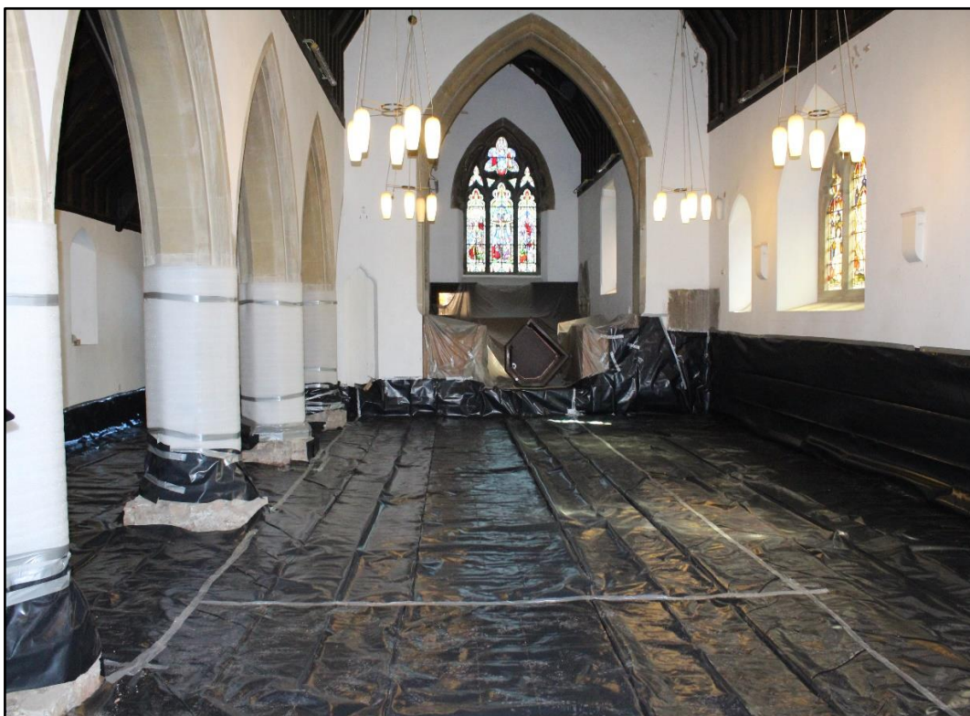
Figure 25: Polythene damp proof membrane laid over the floor area and dressed up walls (Source: Gwynne, 2019).
