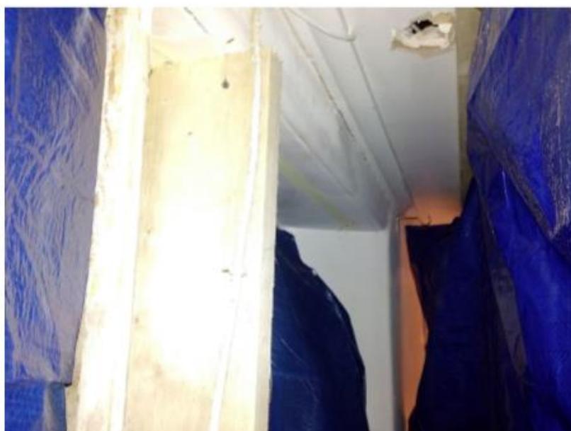
Picture 5 The window frame propped by a short timber stud
