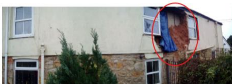
Picture 2 The render above the stonework at ground floor level and the partially collapsed section of the wall.
