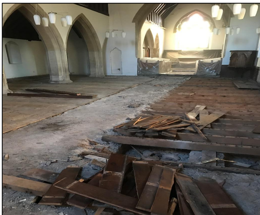
Figure 23: Original ground floor was taken up and removed (Source: Gwynne, 2019).
