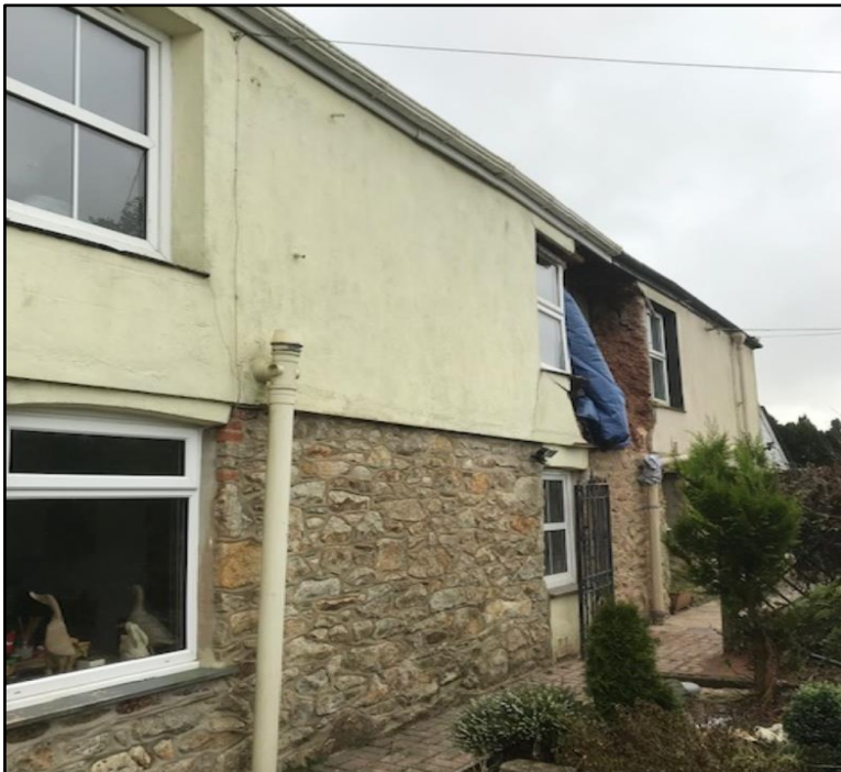
Figure 37: Cob walls renovated with non- permeable finishes
