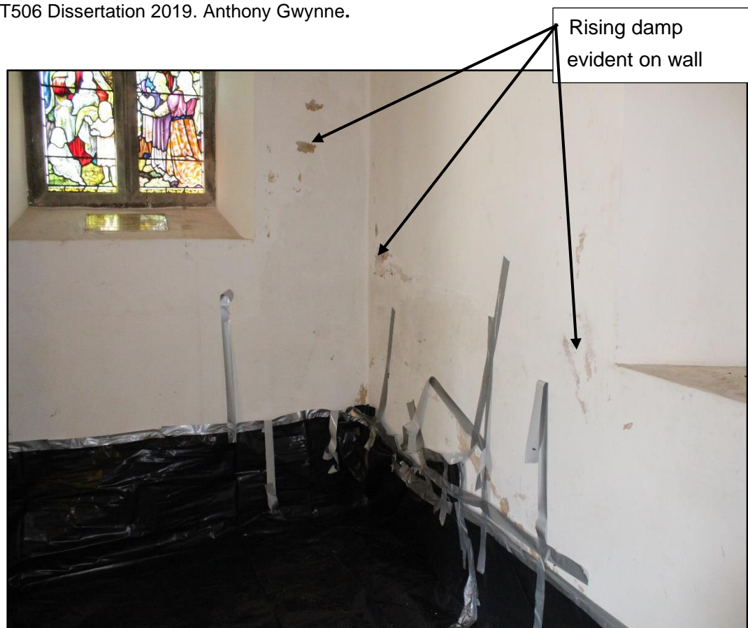
Figure 26: Rising damp evident in walls (Source: Gwynne, 2019).
