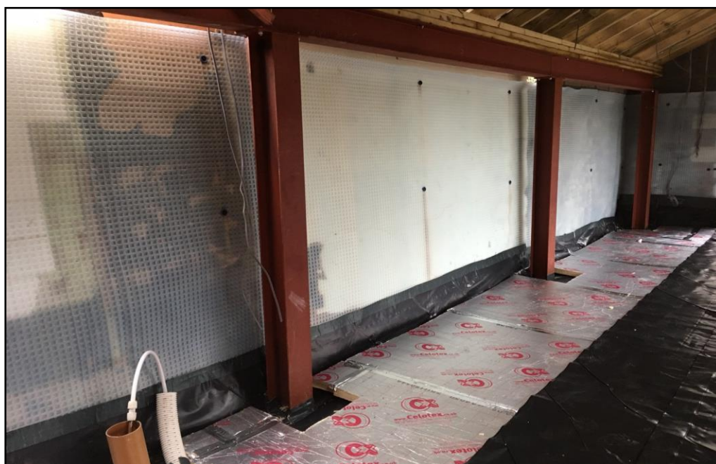
Figure 32: Modern insulation fixed over tanking system ready for concrete floor slab (Source: Gwynne, 2018).
