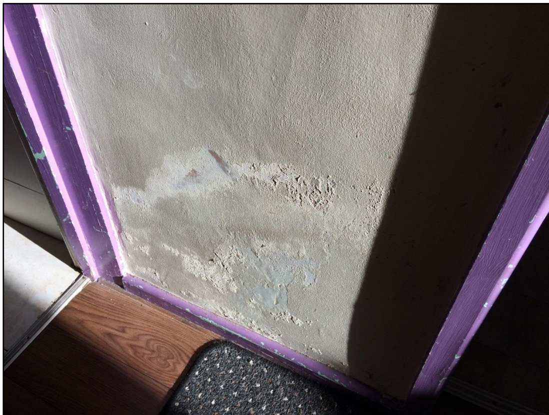
Figure 34: Efflorescence causing damage to hard gypsum plaster and finishes (Source: Gwynne, 2017).
