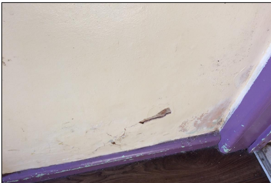
Figure 35: Rising damp and Crypto fluorescence pushing off hard gypsum plaster (Source: Gwynne, 2017).
