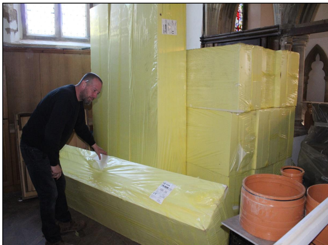
Figure 27: High density polyurethane insulation board 100mm thick was laid over the polythene membrane (Source: Gwynne, 2019).
