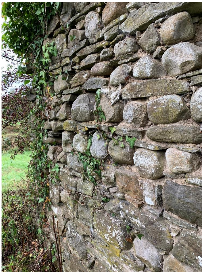
Figure 32 Semi coursed construction of Pant Y Celin. J moriarty.
