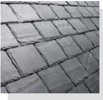
Welsh Slate Roof cladding
