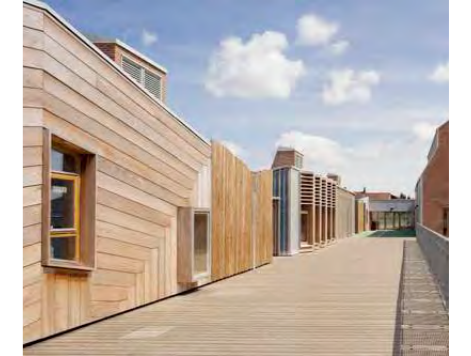
The school uses passive ventilation using brickwork and a ground source heat pump.
