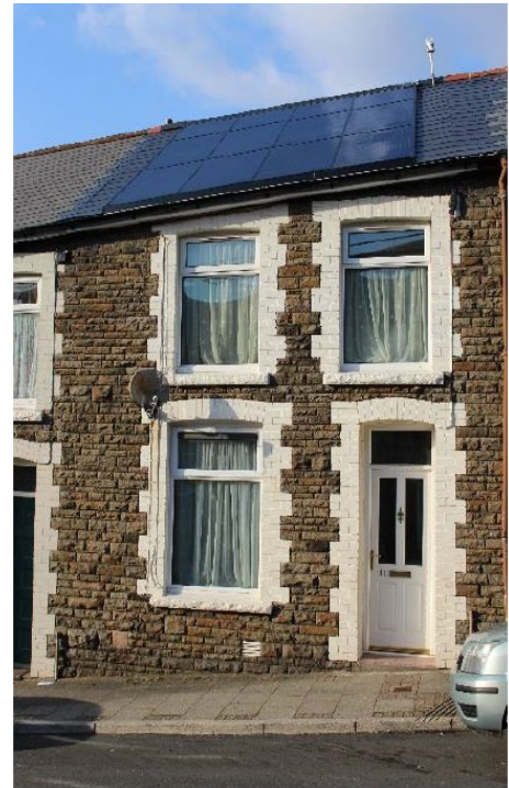
Figure 1. Front House View
